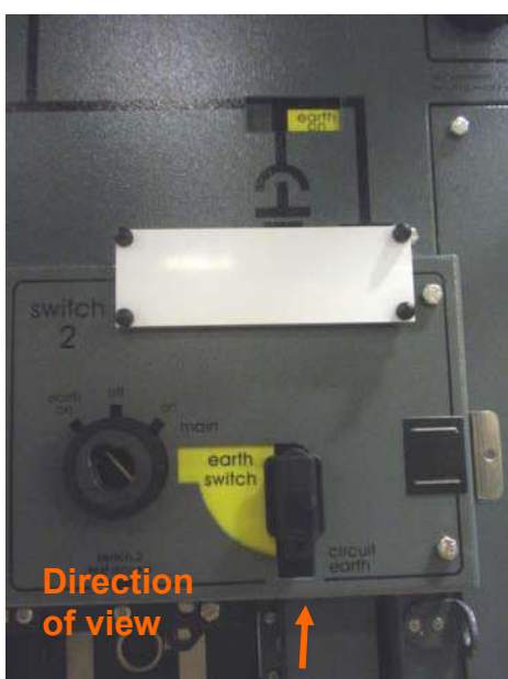
4.20 RSW1 Service position Earth selected Earth ON
