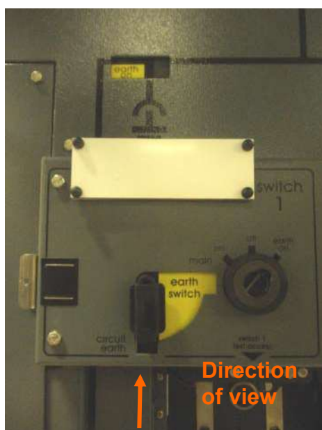
4.20 RSW1 Service position Earth selected Earth ON
