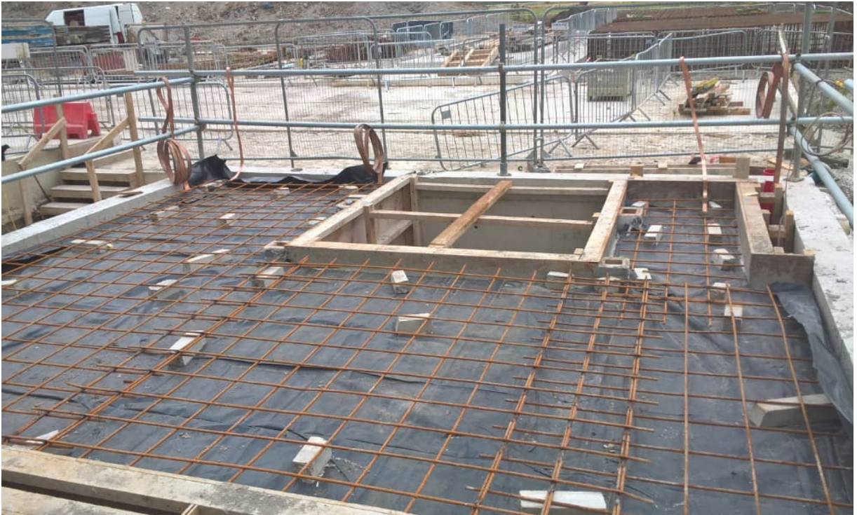
Image 18 – Re-bar flooring with overlap.
