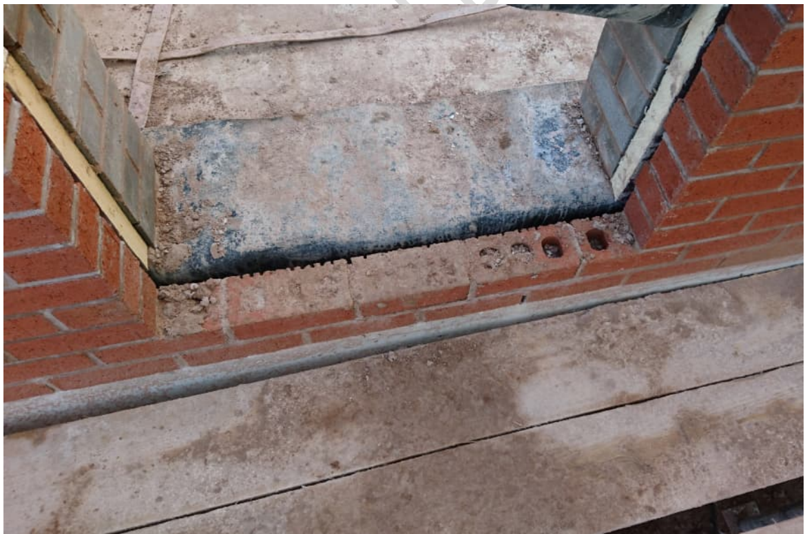
Image 2 - Standard outer brickwork for the entrance to a SPEN substation.
