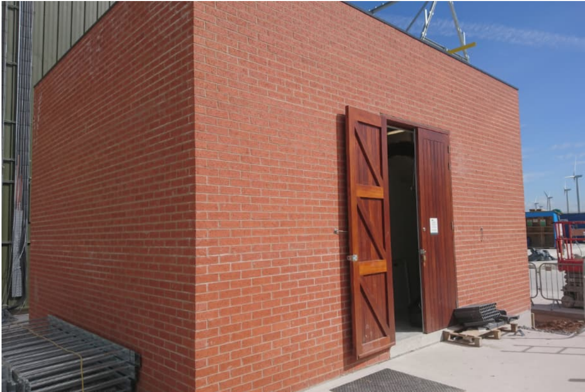
Image 7 – Standard wooden door installed for a SPEN substation.
