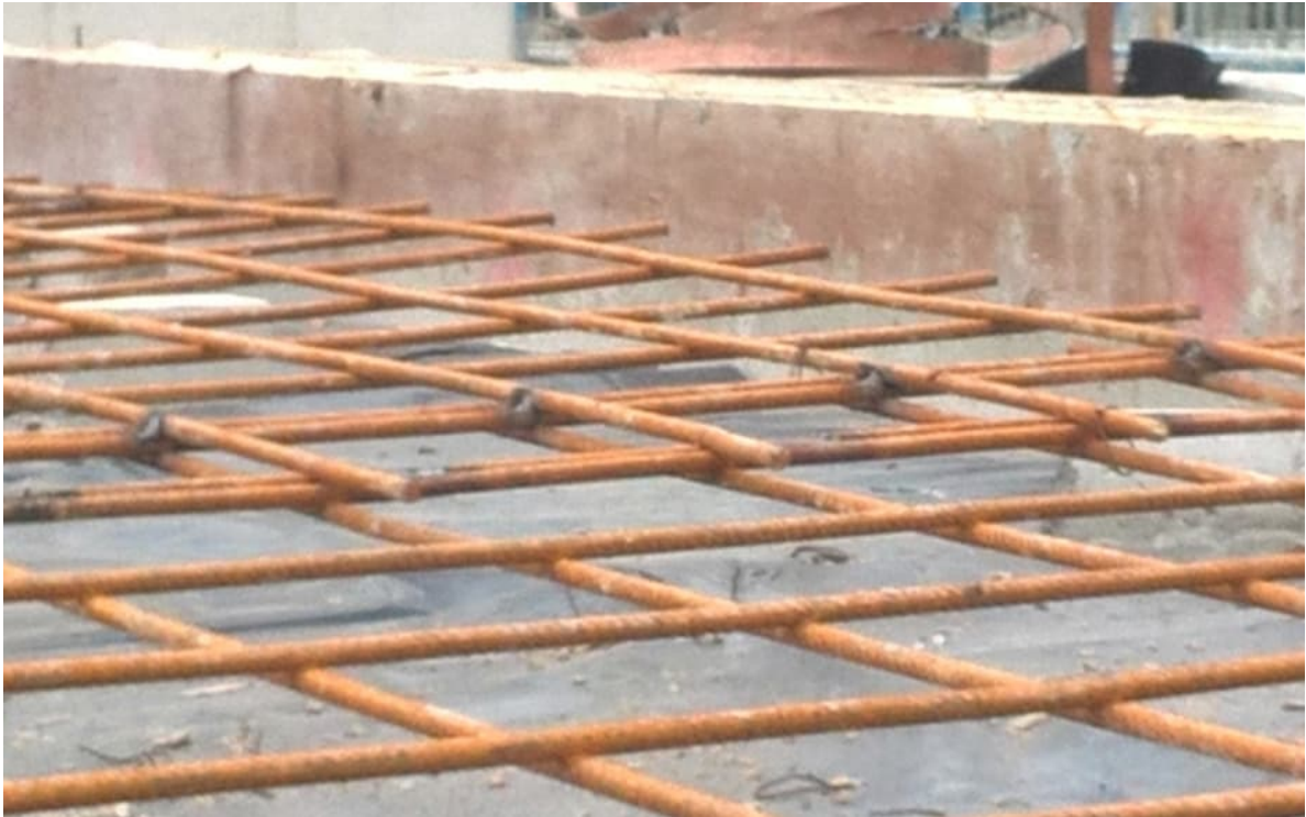
Image 20 – Welded overlap.
