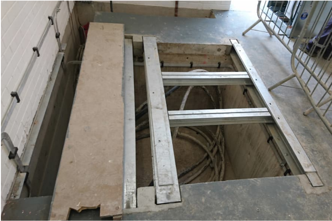
Image 22 - Installation of the steelwork prior to the installation of 3 panel board switchgear (Schneider CBGS-0).
