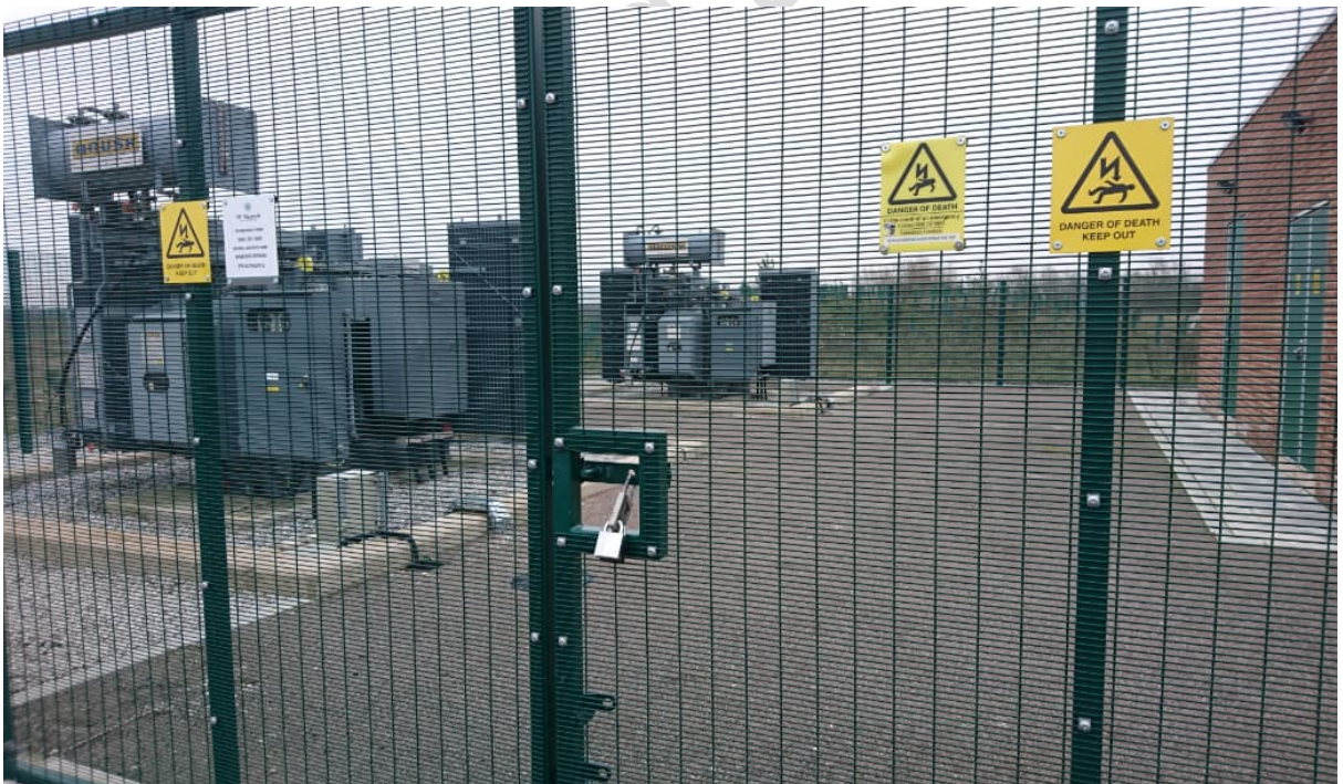
Image 15 – Standard fenced gate with signing and guarding.
