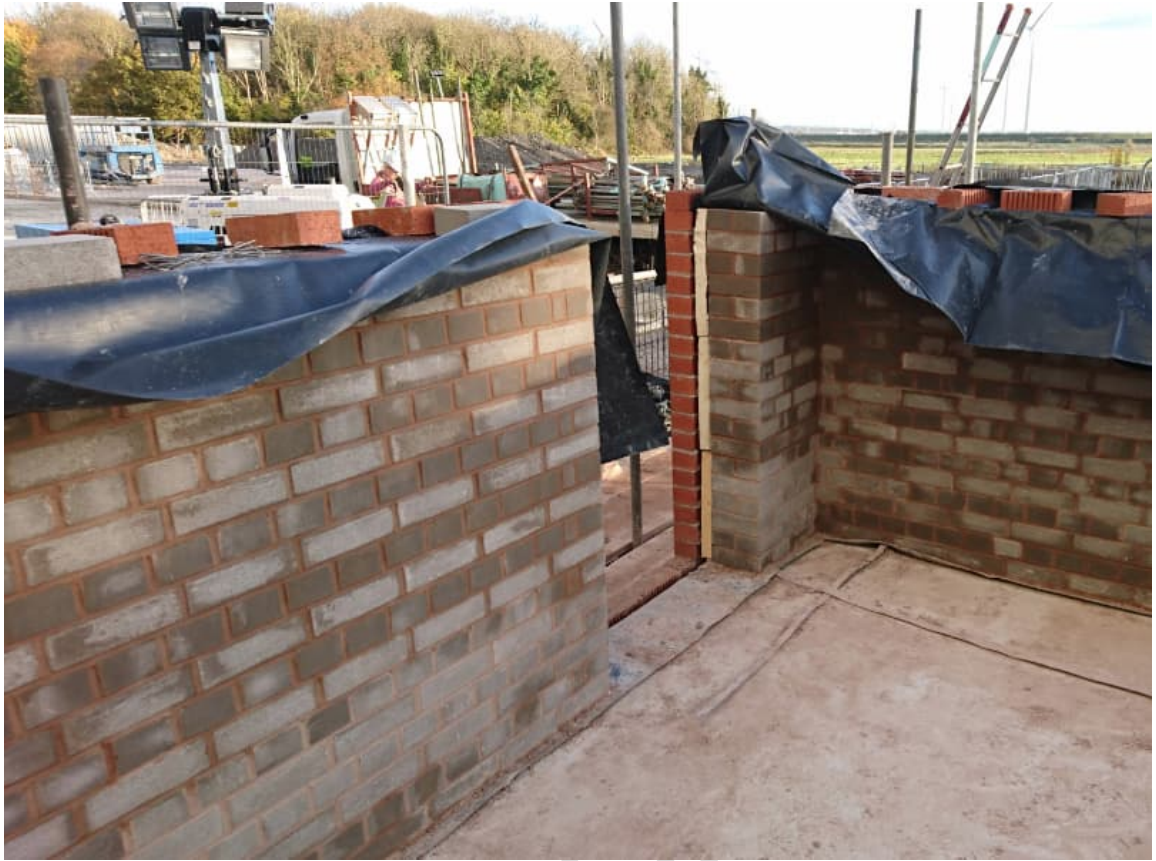
Image 3 - Standard inner brickwork for the entrance to a SPEN substation.
