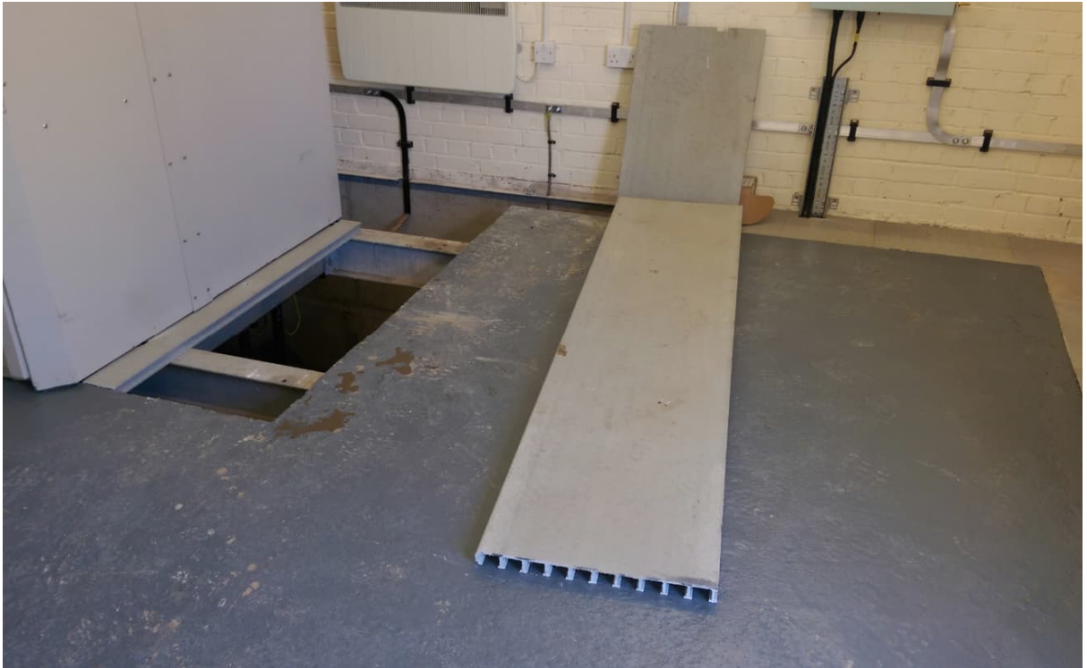
Image 12 – Cable trench cover example.
