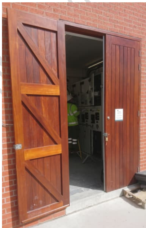
Image 8 – Standard wooden door installed for a SPEN substation.
