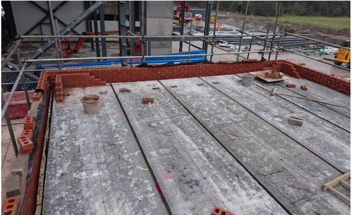
Image 5 – Standard construction of a SPEN substation roof.
