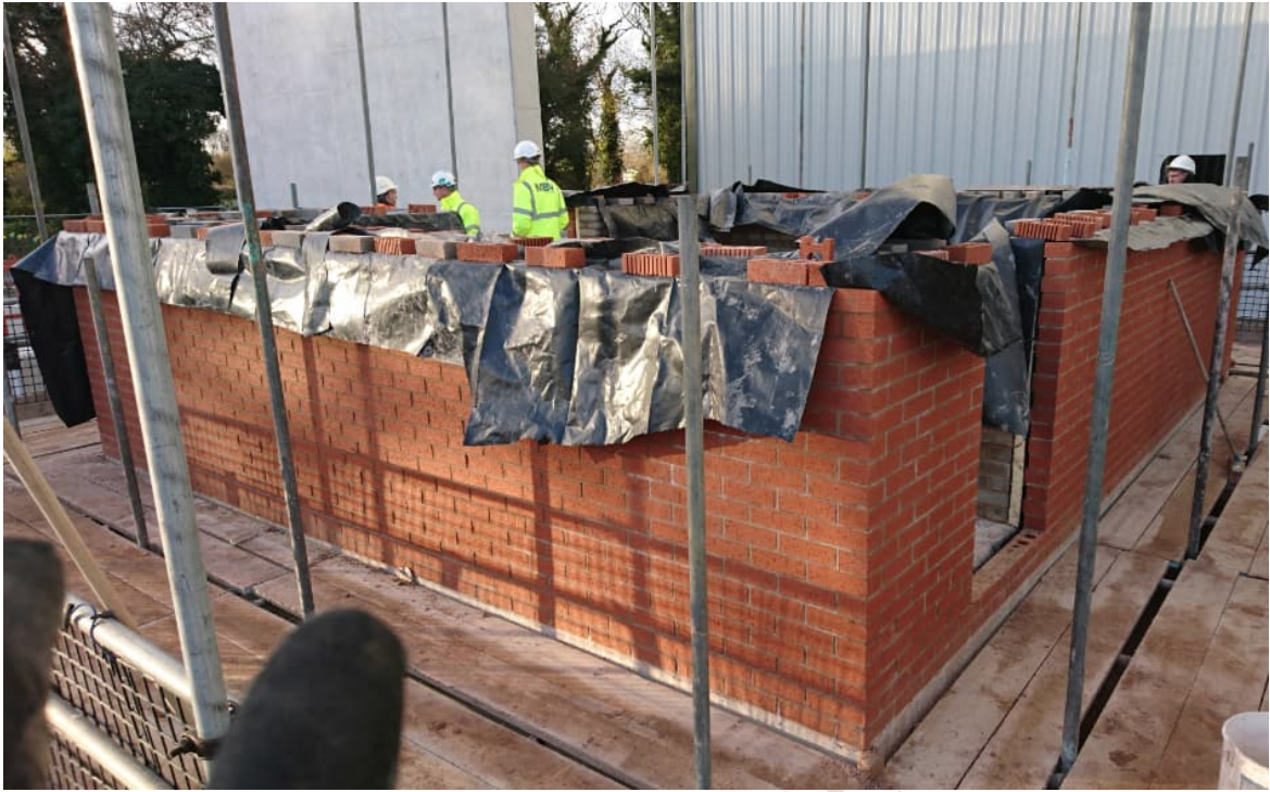
Image 1 – Standard outer brickwork for a SPEN substation.
