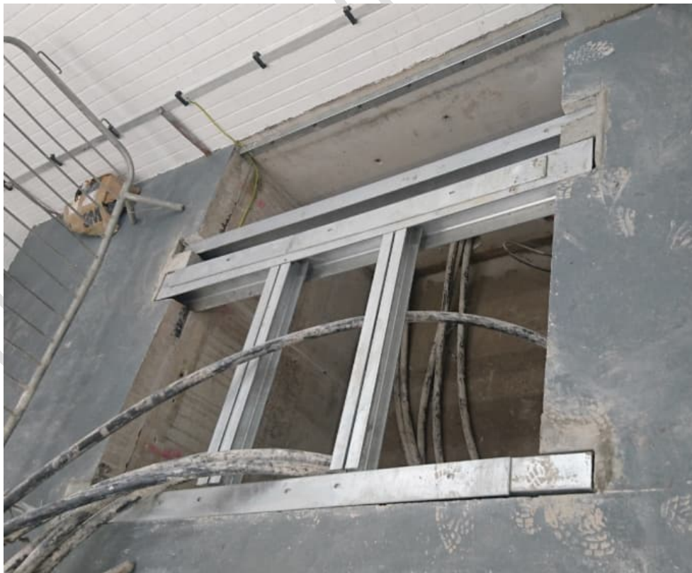
Image 23 - Installation of the steelwork prior to the installation of 3 panel board switchgear (Schneider CBGS-0).
