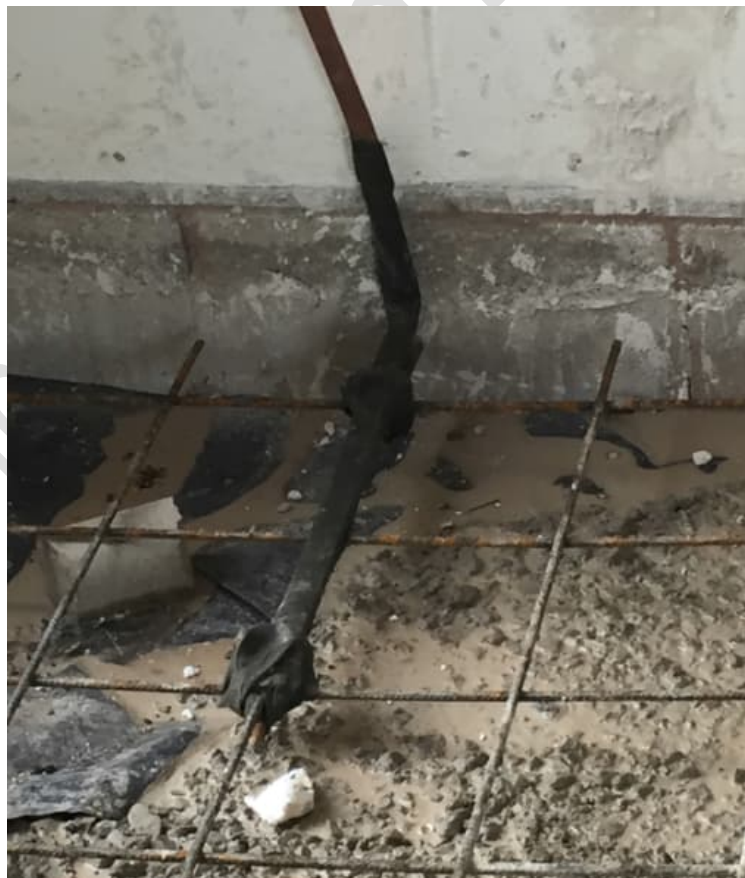
Image 21 – Cad welded earth joint.
