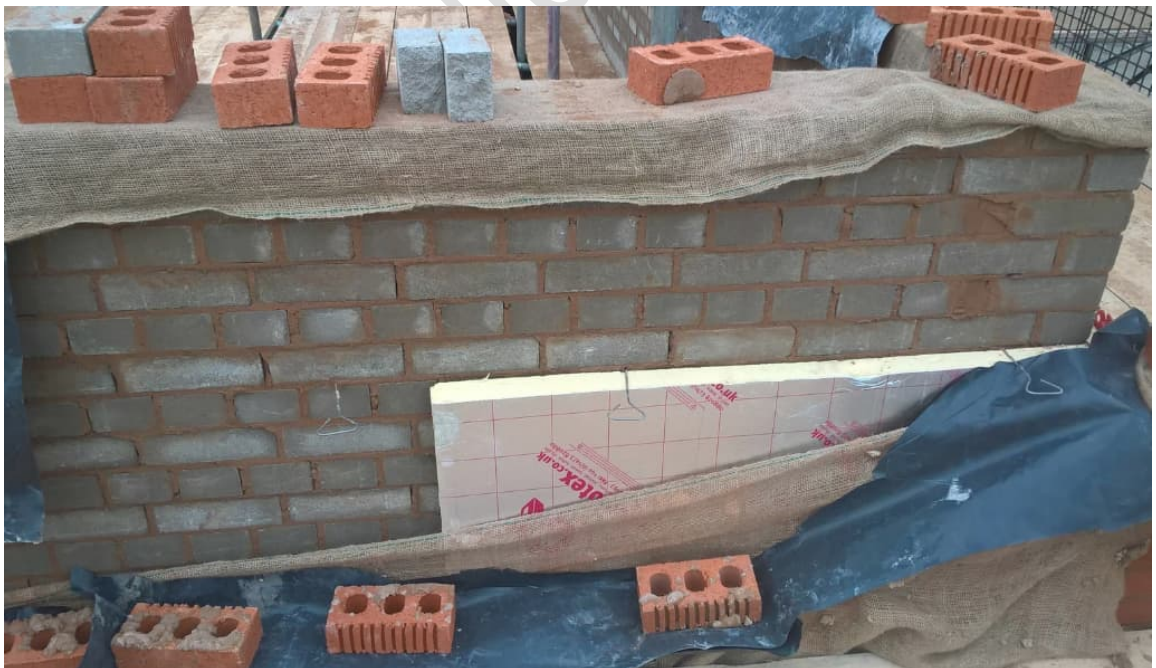
Image 4 - Standard inner brickwork for a SPEN substation.
