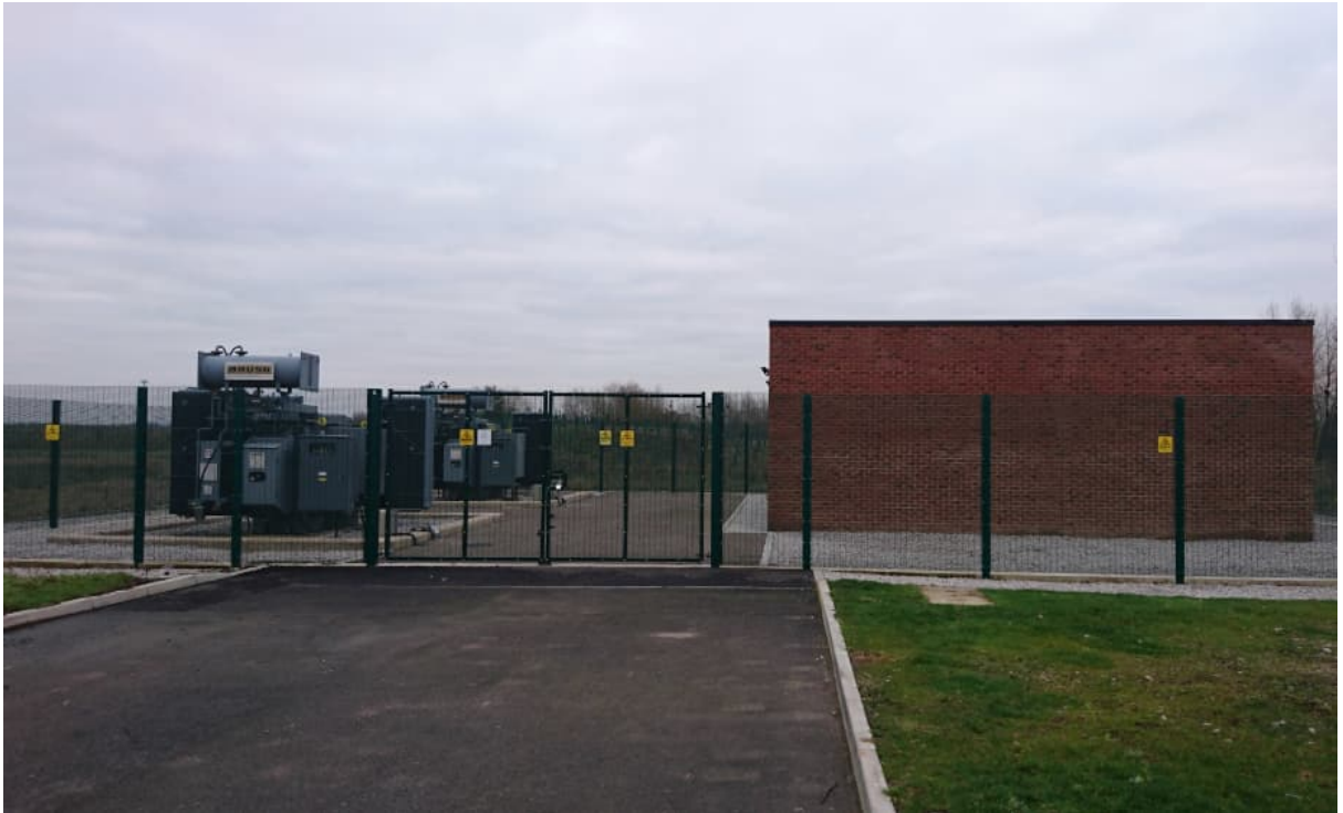
Image 14 – Standard fencing for a substation compound.
