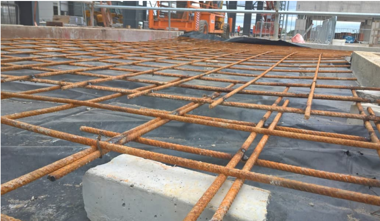
Image 19 - Re-bar flooring with overlap.
