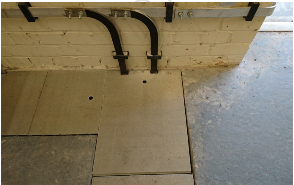
Image 13 – Cable trench cover example.
