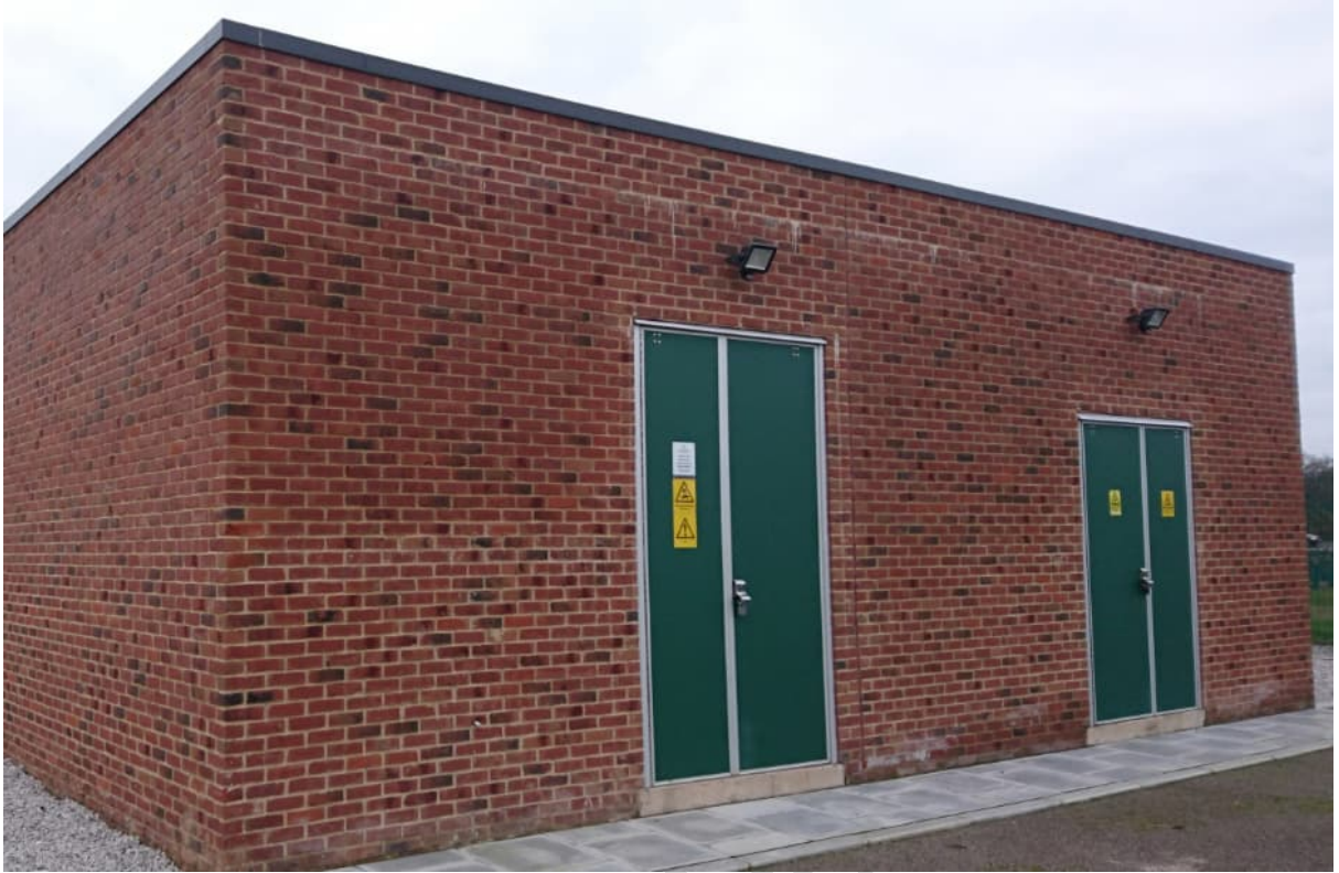
Image 9 - Standard Glass Reinforced Plastic (GRP) door installed for a SPEN substation.
