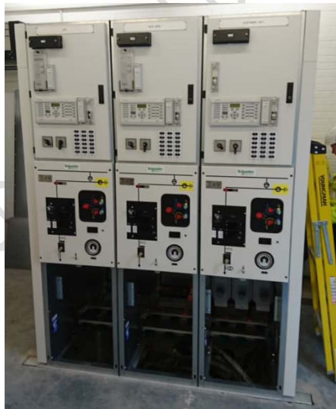
Image 25 – Switchgear Installed.
