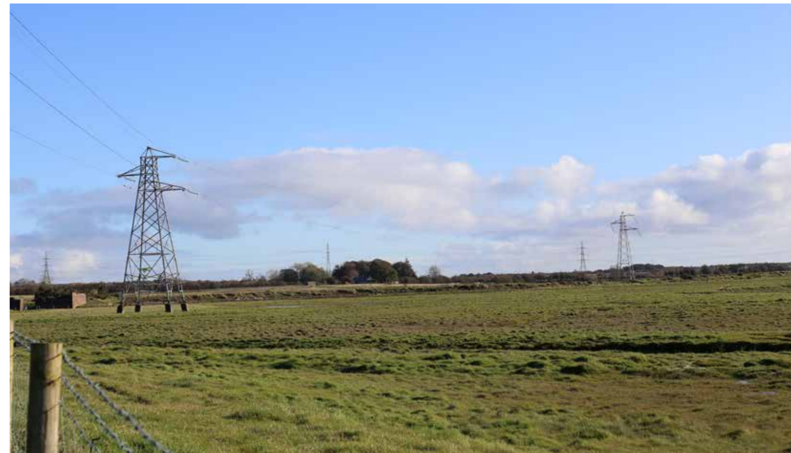
Photo 2: Existing steel towers of T Route
