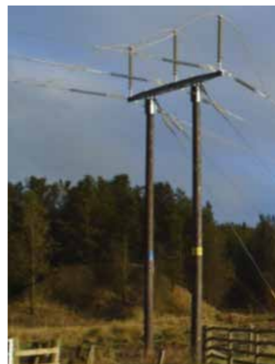
Photo 5: Typical H Pole
