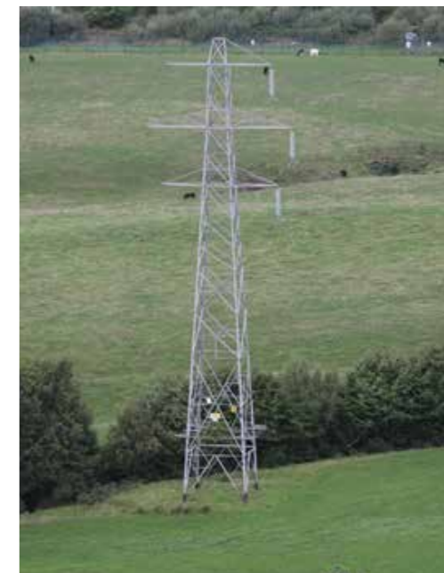
Photo 6: Single Circuit Steel Lattice Tower with conductors only on one side
