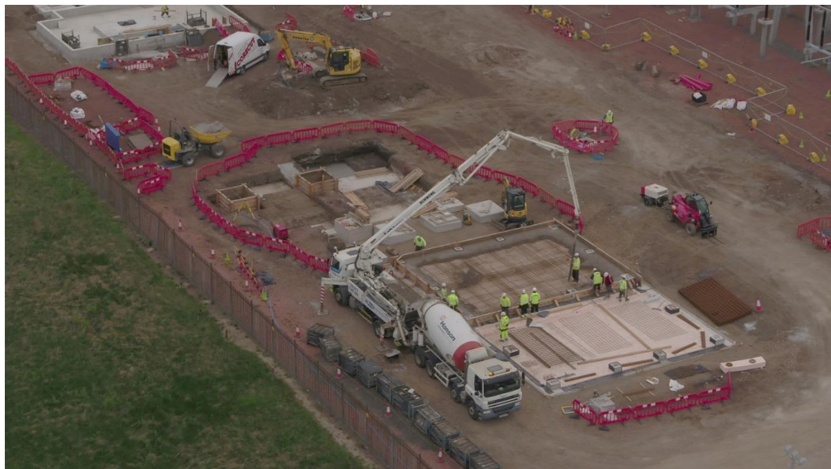
Figure 2 – STATCOM Base being poured
