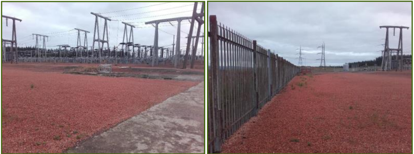
Figure 7 – Photographs from Site Visit
