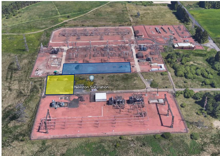
Figure 6 – Phoenix Installation Site, showing CDM Welfare Area (marked in yellow)
