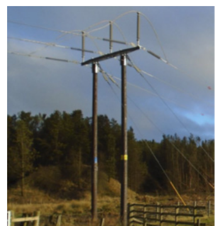
Typical double wood 'H Pole'
