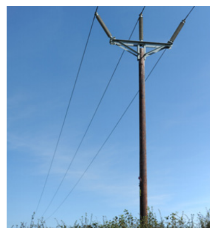
Typical Trident single wood pole
