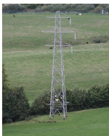
Single circuit steel lattice tower
