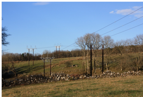
Double 'H' Pole 132kV Overhead Line
