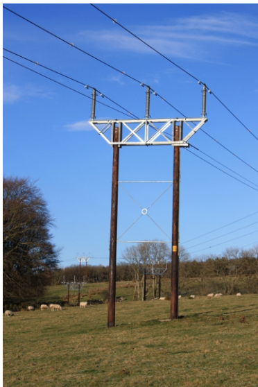
Double 'H' Pole 132kV Overhead Line
