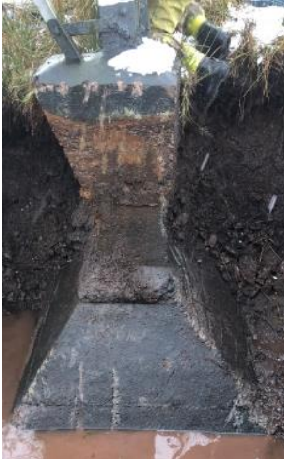
BW016 Tower Foundation
