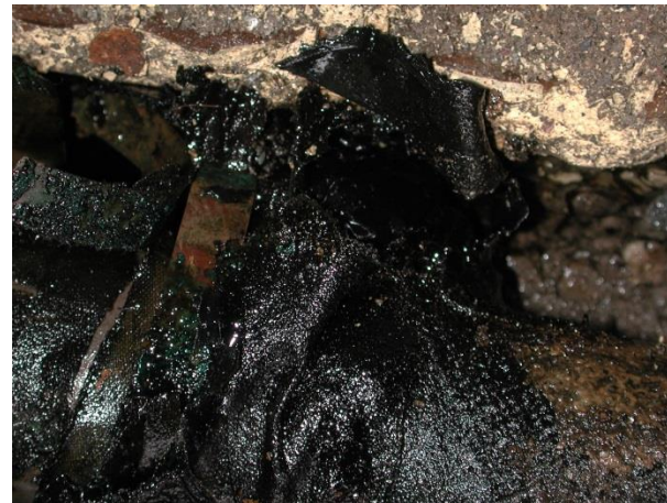
Figure 4: Damage in [REDACTED] 2011. (Gorgie-Telford Road circuit)
