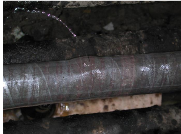
Figure 2: 2011 Cable Prepared Ready for Repair. (Gorgie-Telford Road circuit)
