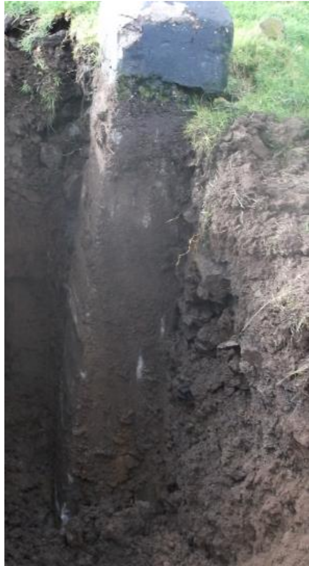
AY019 Tower Foundation: absence of pyramid AY027 Tower Foundation: absence of pyramid
