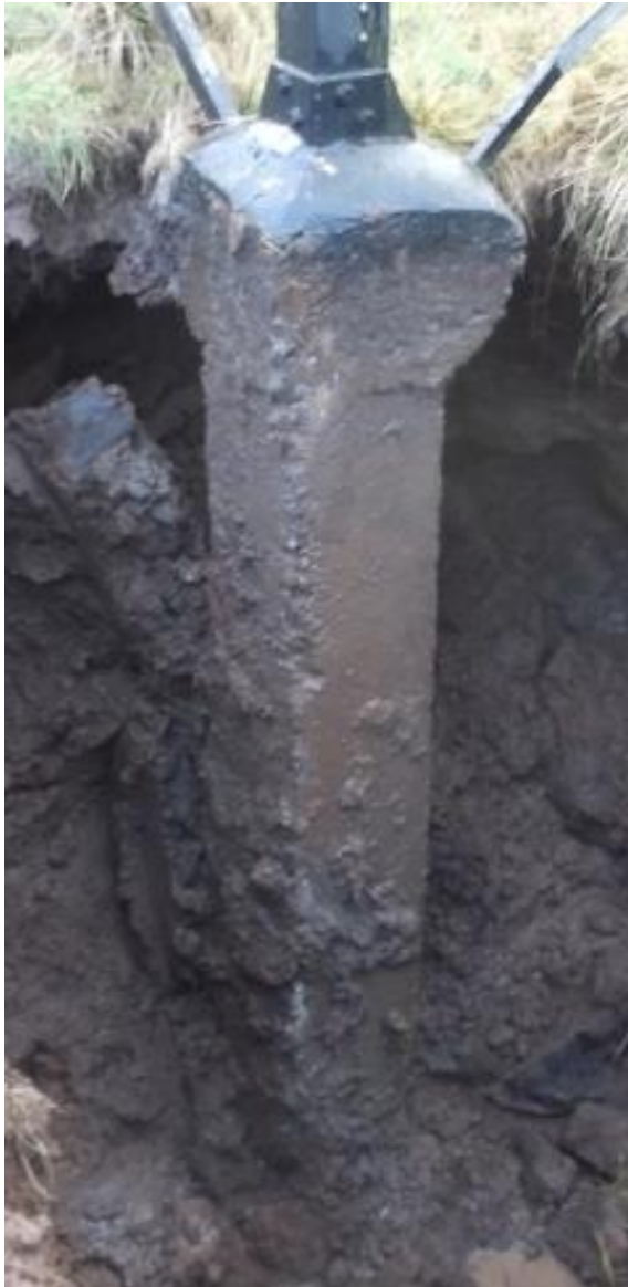
AY019 Tower Foundation: absence of pyramid AY027 Tower Foundation: absence of pyramid
