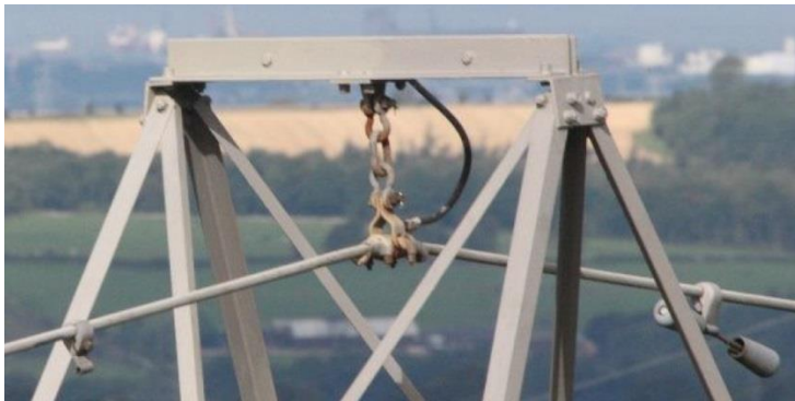
Figure 3 & 4: earth wire fittings worn, dampers collapsed and broken and insulators strings showing rust and missing discs.
