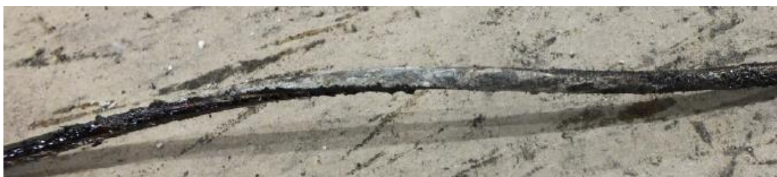
Figure 2: steel core strands exhibiting rusting.
