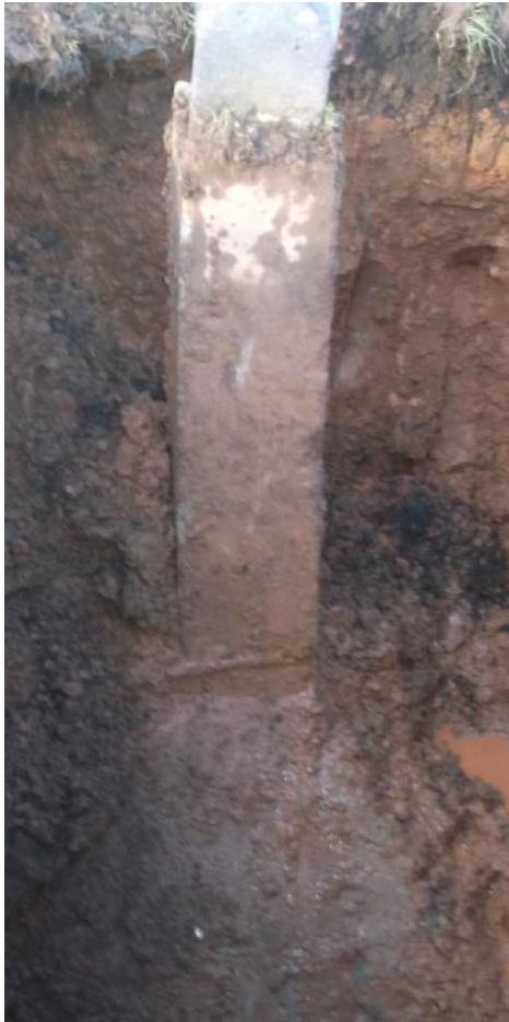
AL043 Tower Foundation
