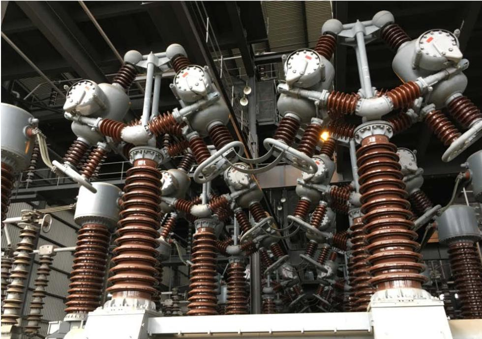
*Figure 2: OIBR80 circuit-breakers at Longannet 275kV substation*
