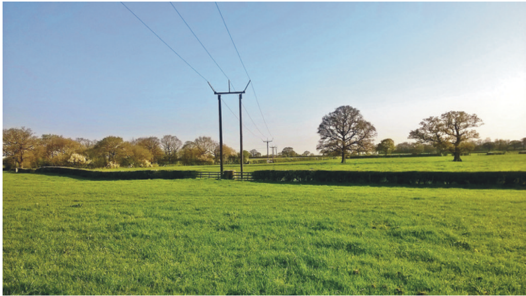
Typical 132kV Trident wood pole overhead line design with “H” pole in foreground and Single pole behind.
