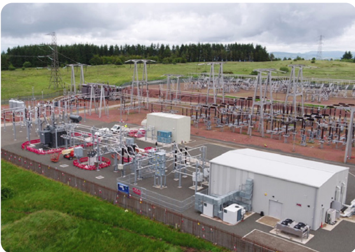
Phoenix Project at Neilston Substation
