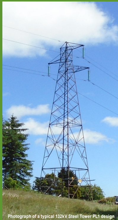
Photograph of a typical 132kV Steel Tower PL1 design
