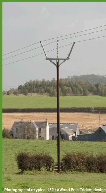
Photograph of a typical 132kV Wood Pole Trident design
