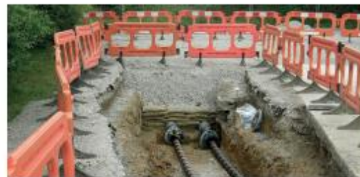
Underground cable installation during construction
