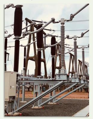
Figure 17 Optical instrument transformers installed at Wishaw 275kV substation (project FITNESS)
