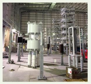
Figure 31 Harmonic Filters at Western HVDC converter station
