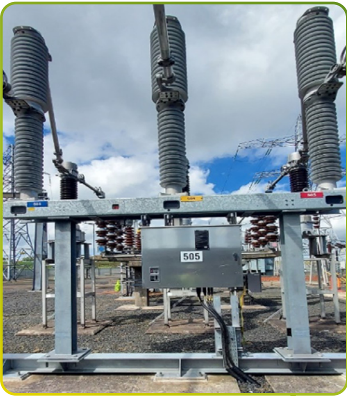
Kilwinning and Meadowhead Circuit Breaker changes, removing aging SF 6 Assets and installing new Clean Air CB's from Siemens.
