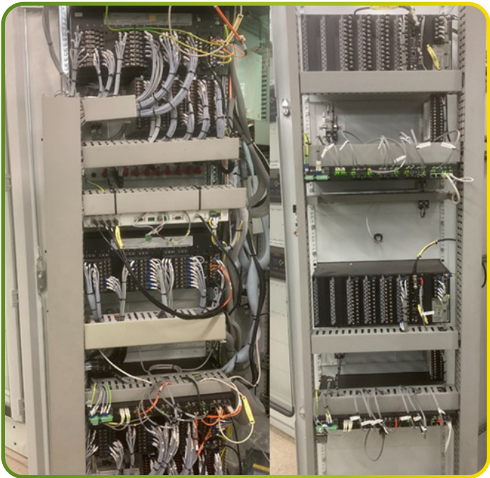
Comparison of conventionally wired panel (West Coast Operational Intertrip Controller Panel at STHA4 on left vs ASACS Controller panel at STHA4 on right).
