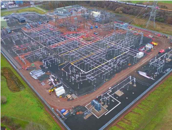
Wishaw 275kV Substation
