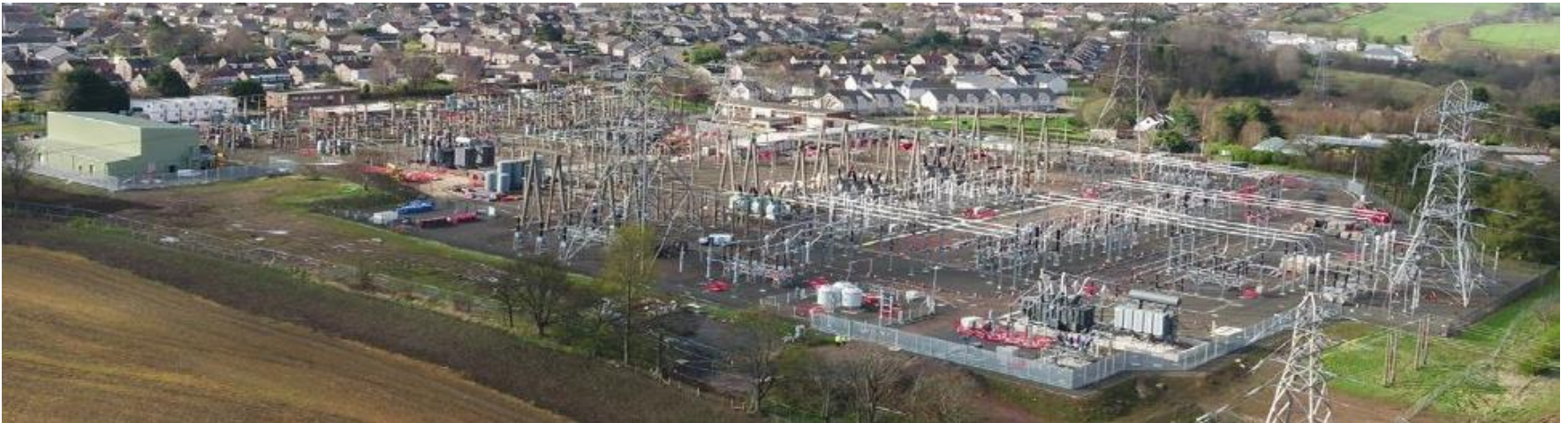
Currie 275/132kV Substation
