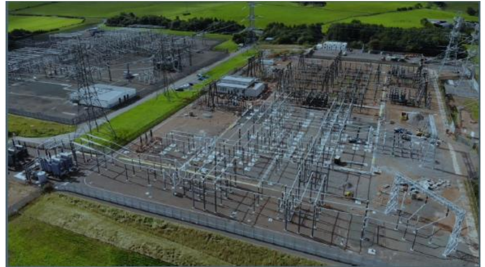
Strathaven 275kV Substation
