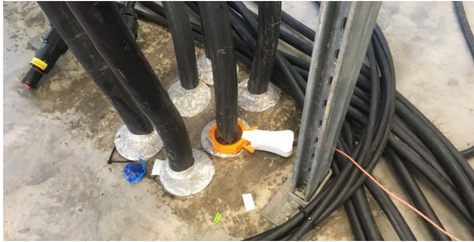
HV/LV Device being tested at the Power Networks Demonstration Centre
