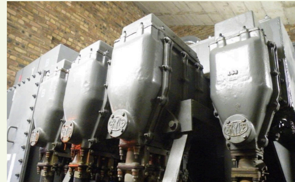
G38 Units with signs of leakage
