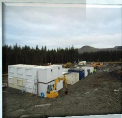
Work underway at the substation location includes the installation of a site compound with temporary offices. Work has also started to clear and level the area that will create the concrete platform. This platform will provide the base for the substation and house the mechanical and electrical infrastructure to be installed.
