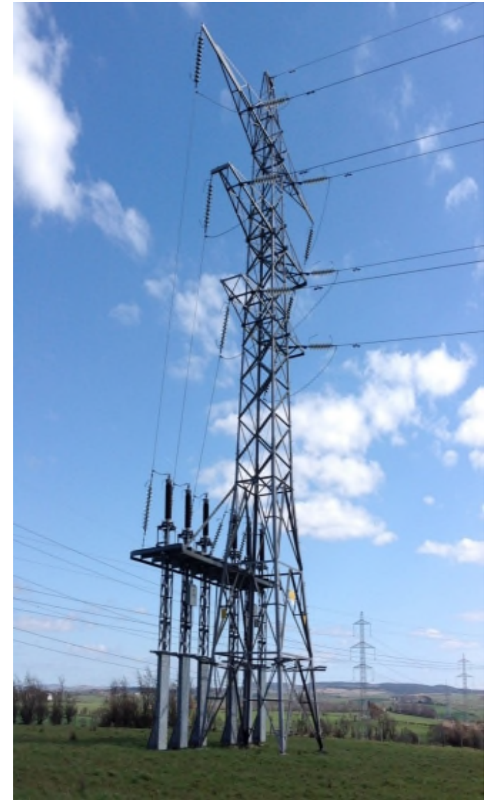
Sealing end tower south of Coylton substation
