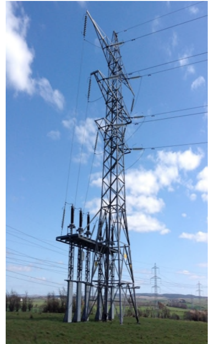
Sealing end tower south of Coylton substation
