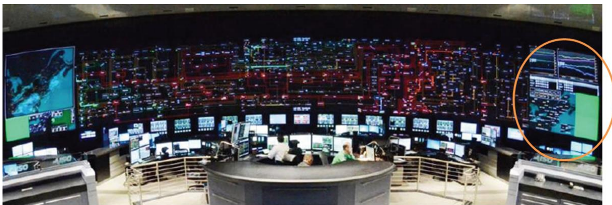
Figure 12. Example of WAMS system used on the NYISO control centre video wall (encircled) 2
