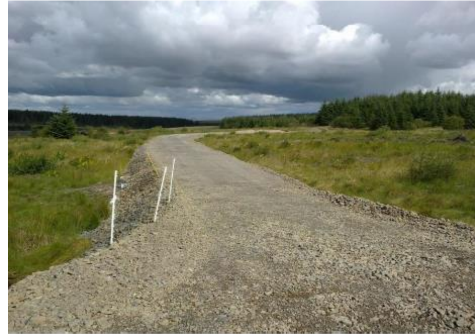
Photo 4.7 (a) and (b): Stone Tracks – Floating Tracks (B2)
