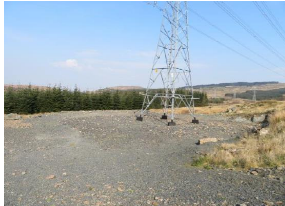
Photo 4.9: Typical Working Area
