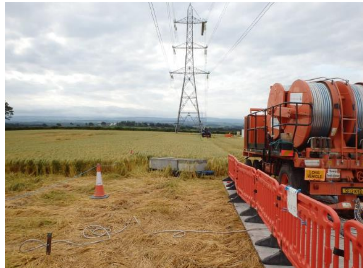
Photo 4.11: Stringing of Steel Tower
