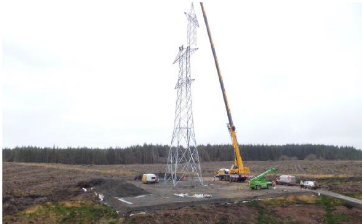
Photo 4.10: Typical Working Area
