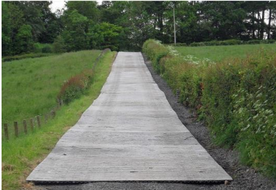
Photo 4.8 (a) and (b): Plastic and Aluminium Matting (C)
