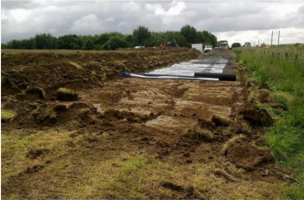
Photo 4.6 (a) and (b): Stone Tracks – Cut and Fill Tracks (B1)
