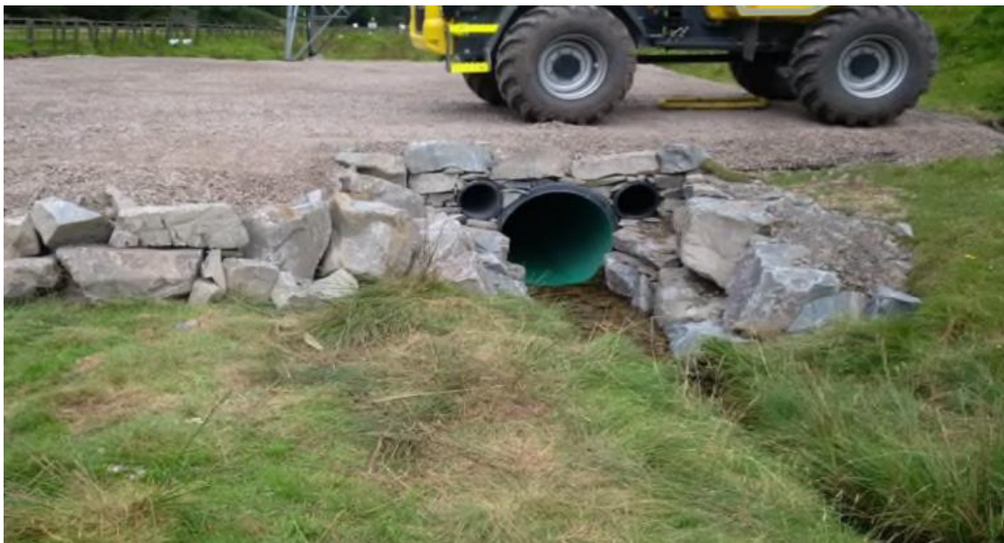
Photo 3.6 Typical Culvert Crossing
