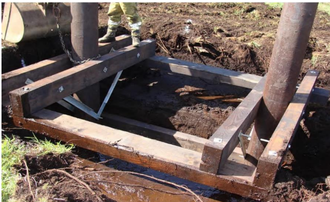
Photo 3.9 Foundation Bog-shoe Arrangement for Poor Ground Conditions
