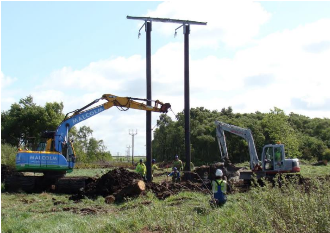
Photo 3.8 Pole Installation by a Track Excavator
