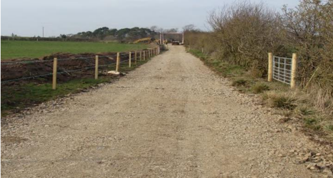
Photo 3.4 Typical Stone Temporary Access Track
