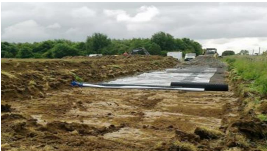
Photo 3.3 Temporary Access Track Installation Using Geomembrane
