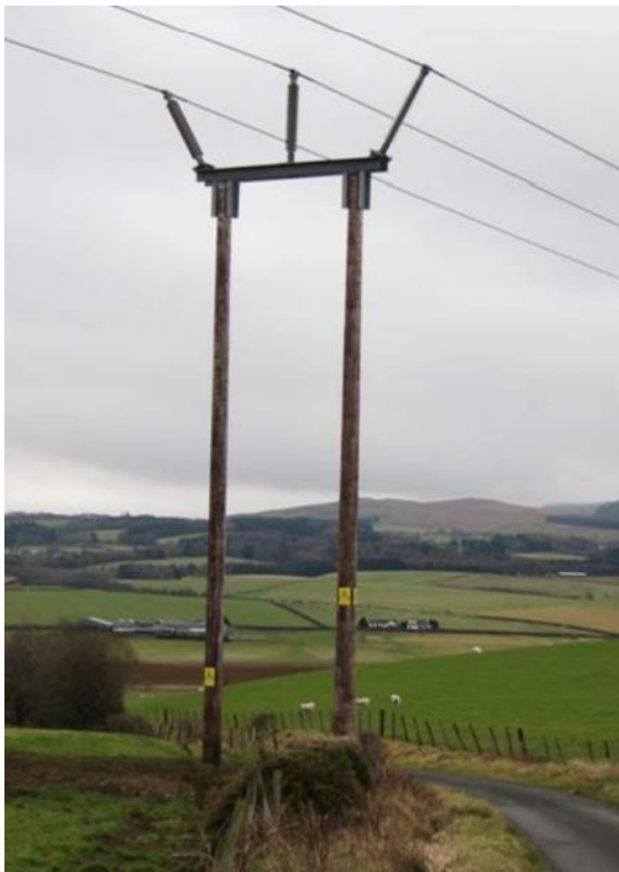
Photo 3.1 Typical Intermediate H Pole
