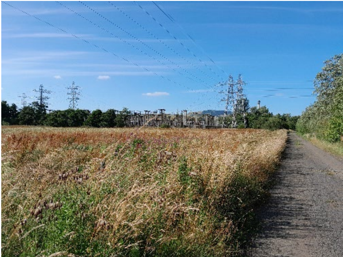
Image 3.6: Westfield Substation View from the South-East.
