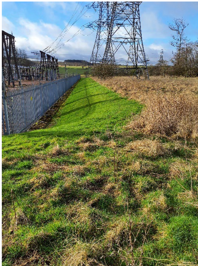
Image 3.5: Westfield Substation Western Boundary.
