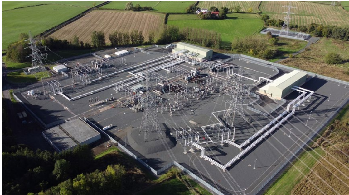
Image 2.1: Example of an existing substation.
