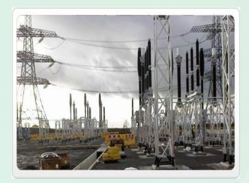
The formation of the overhead line towers will see concrete foundations being laid, these involve deep foundation concrete piles being delivered to the site during the first half of 2014, once installed steel lattice towers will be erected in sections. It is intended that this phase of construction will be completed by late 2014.
