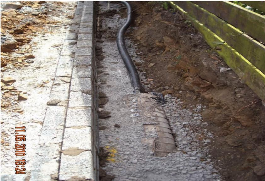
The above image highlights a situation which occurs all too frequently, no cable records or cable locator on site, customer in the process of constructing a garage damages a distribution cable.
