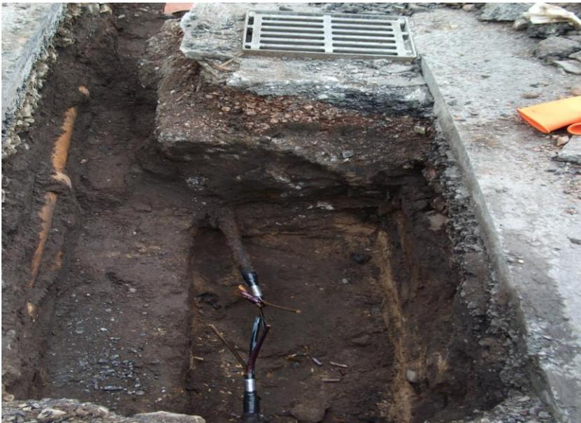
The above image demonstrates a low voltage cable fault on ScottishPower's underground electrical network.
