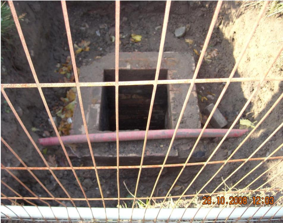
The above image highlights a situation where a ScottishPower high voltage cable was found to be constructed into a drainage manhole.
