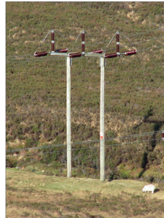
Trident 'H' pole straight-line pole
