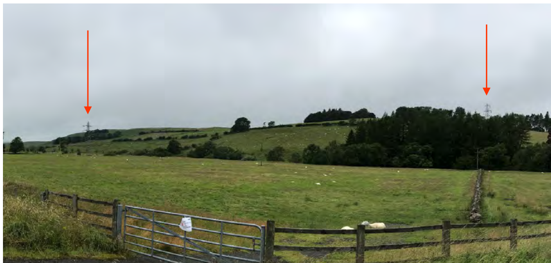
Image 7.5: Potential V-Route Connection Towers
