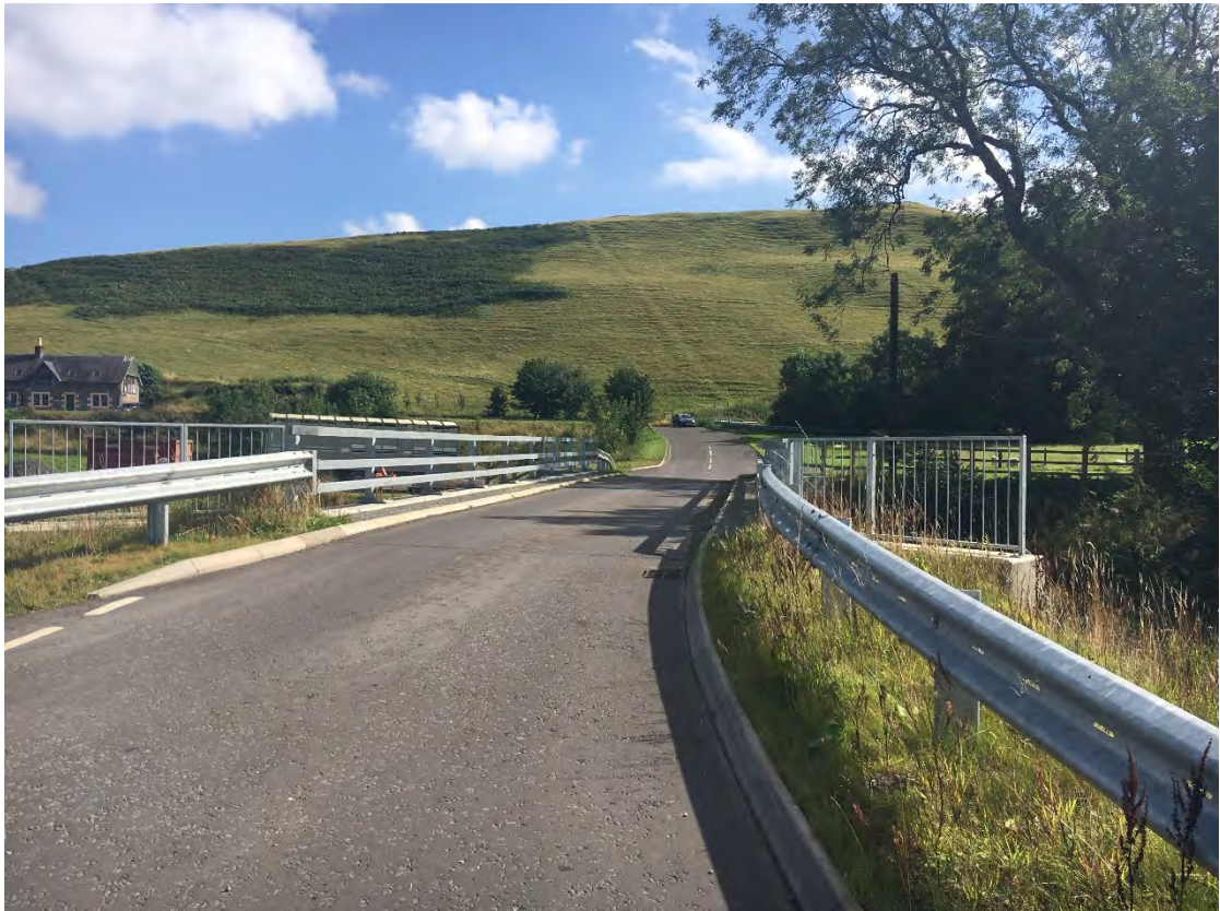
Image 6.9: Photo Point A – View of Falnash Burn Road from A7
