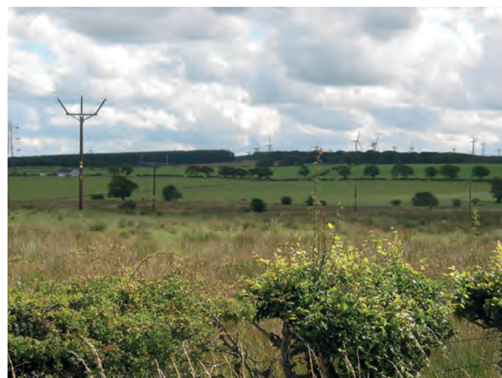
Trident single poles in lowland setting, with wind farm
