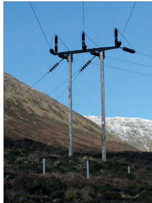
Trident 'H' pole turning pole
