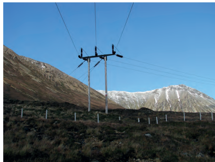
Trident 'H' turning pole in moorland setting
