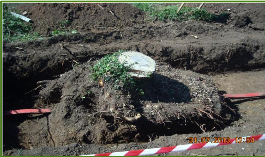
The above image demonstrates a situation where a tree has been installed on top of a high voltage cable. The task for the contractors was to remove the tree stump to enable drainage pipes to be installed beneath the cable with a view to also forming a new carriageway entrance in the future.
