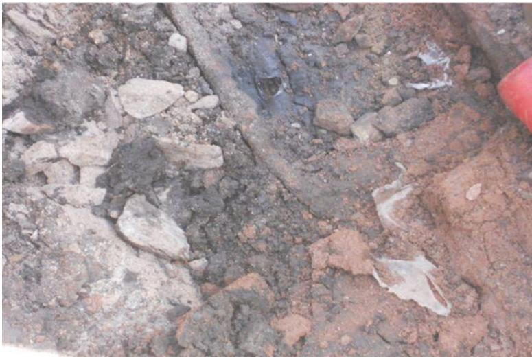
**The above image highlights a low voltage cable strike to the ScottishPower electrical network.**
