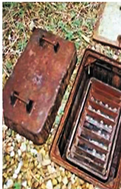
The above images highlight low voltage underground switching boxes (link boxes) protected with a concrete cover.
