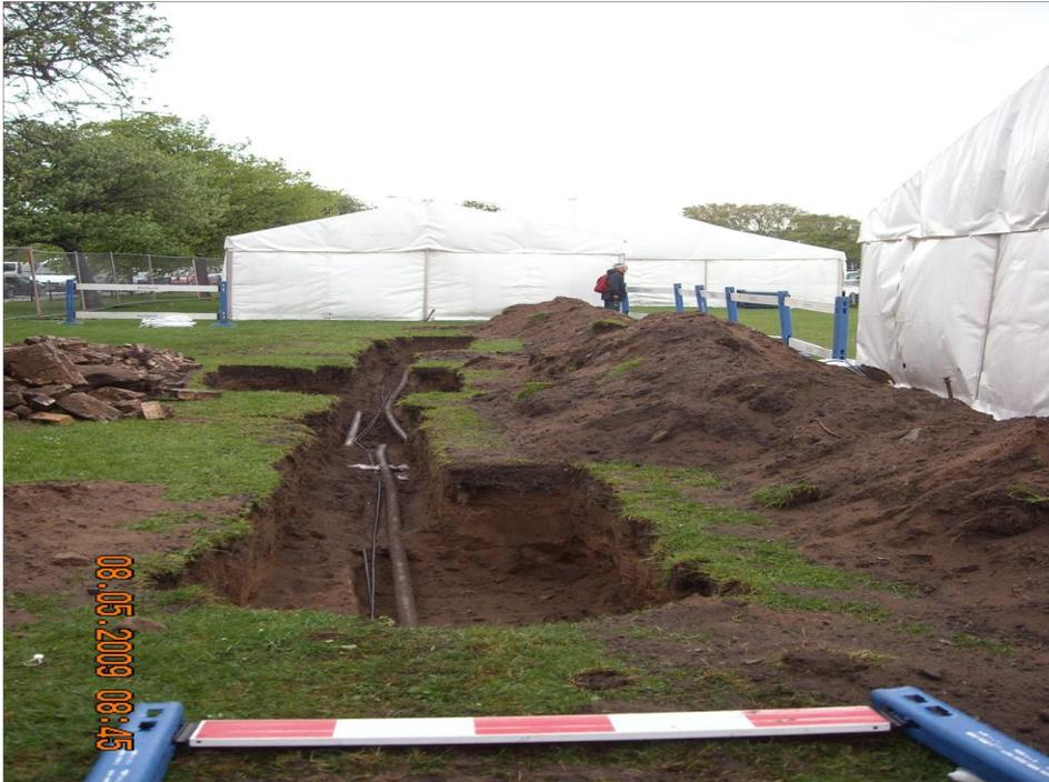
The above image highlights a situation when a high voltage cable was damaged when a 910mm long steel pin was driven into the ground whilst erecting a marquee. This example demonstrates the impact on the ScottishPower network due to poor implementation of safe working practices. On this occasion no ScottishPower cable records or cable avoidance tool on site. Please contact ScottishPower cable records prior to commencing any work..
