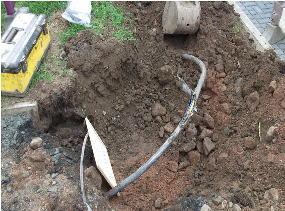
**The above image highlights the consequences of utilising a mini excavator in close proximity to a low voltage cable.**
