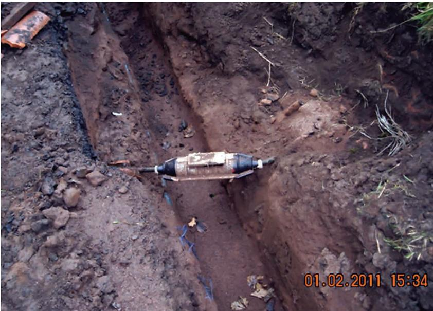
The above image highlights a repair to a ScottishPower low voltage service cable.
