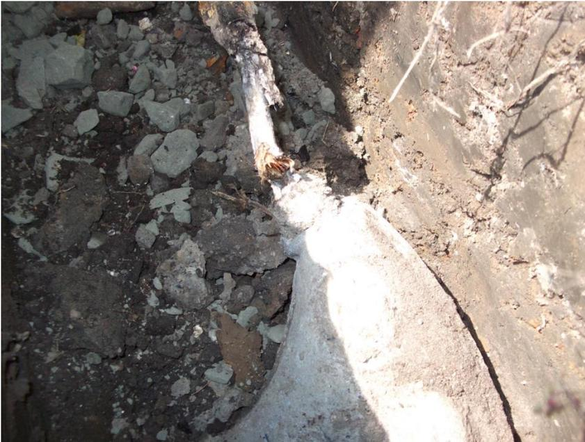
The above image highlights a low voltage cable strike to ScottishPower's underground electrical network.
