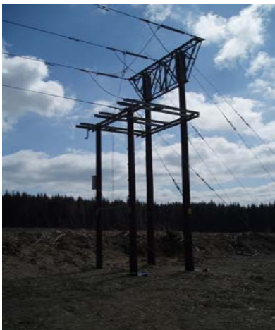
7. Terminal (4 pole) structure; with stays
