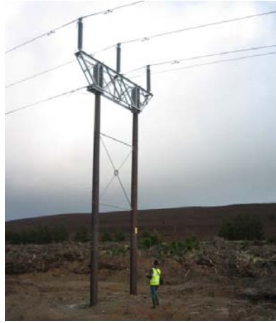
2. H pole support type used in straight line situations
