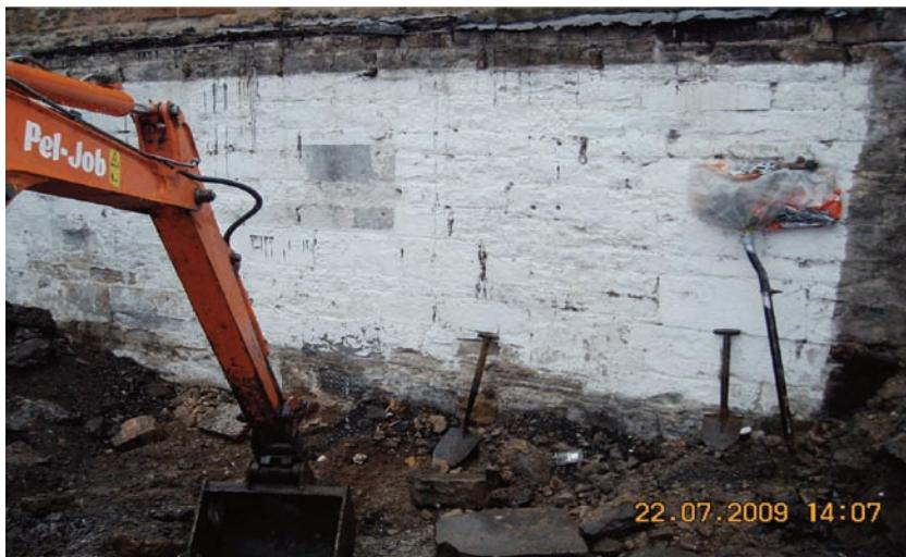
The above image highlights a situation where a garage was in the process of being demolished, exposing a live electrical cable head covered with a plastic bag.
