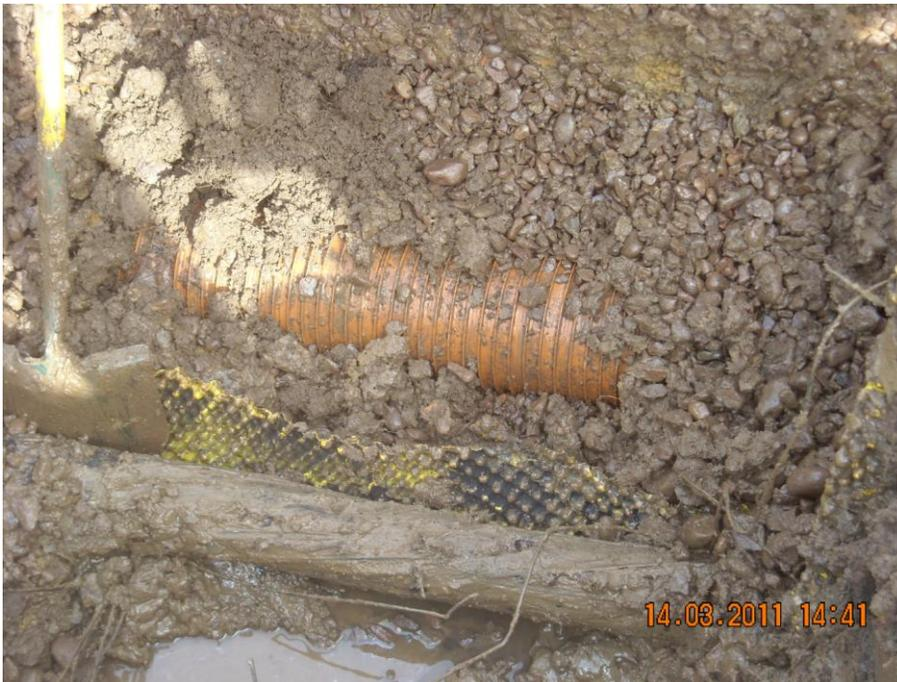
The above image highlights the consequences of lack of separation between ScottishPowers 33KV wired armoured cable and the newly installed field drain
