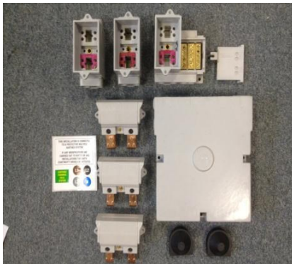
Example of insulated cut-out that can be changed using this procedure
