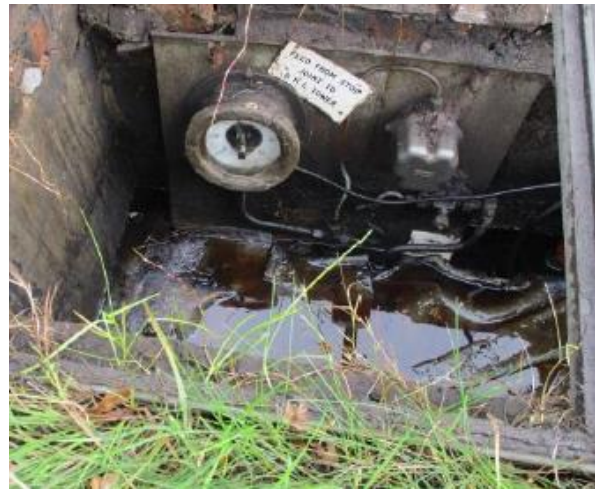
Figure 4: condition of Greenock road stop joint gauge.
