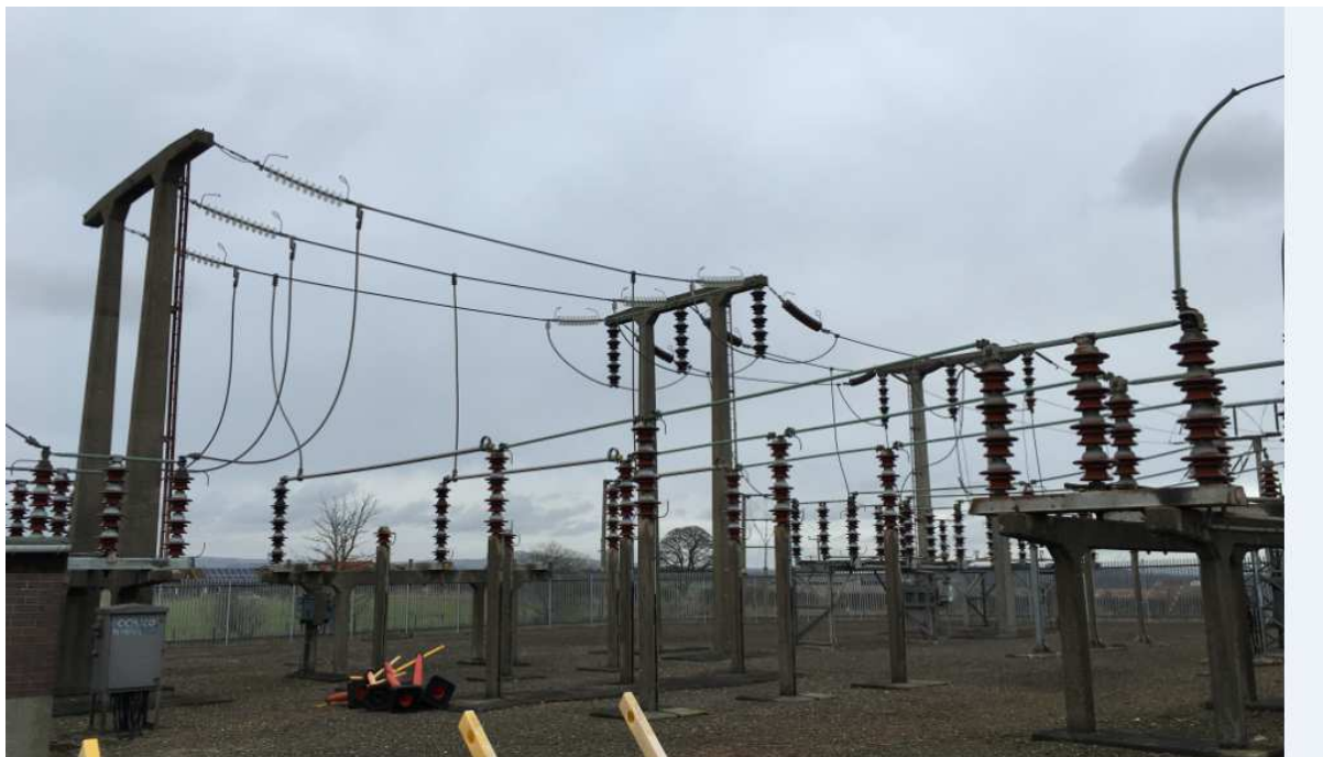
Figure 2: Existing concrete gantries proposed to be reused at Glenniston 132kV substation
